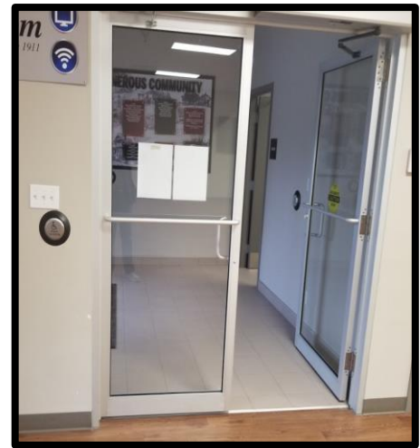
Figure 7: Push Button for Exit
