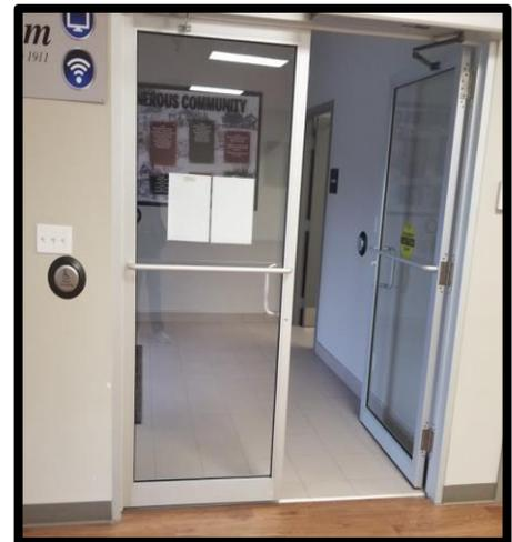
**Figure 7: Push Button for Exit**
